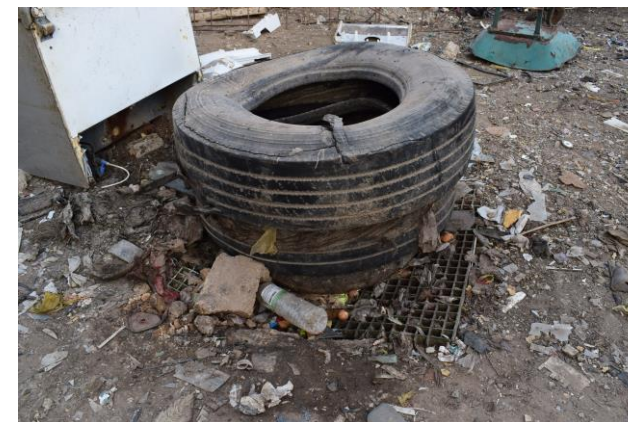
Regard obstrué (Photo USF, 2018)
